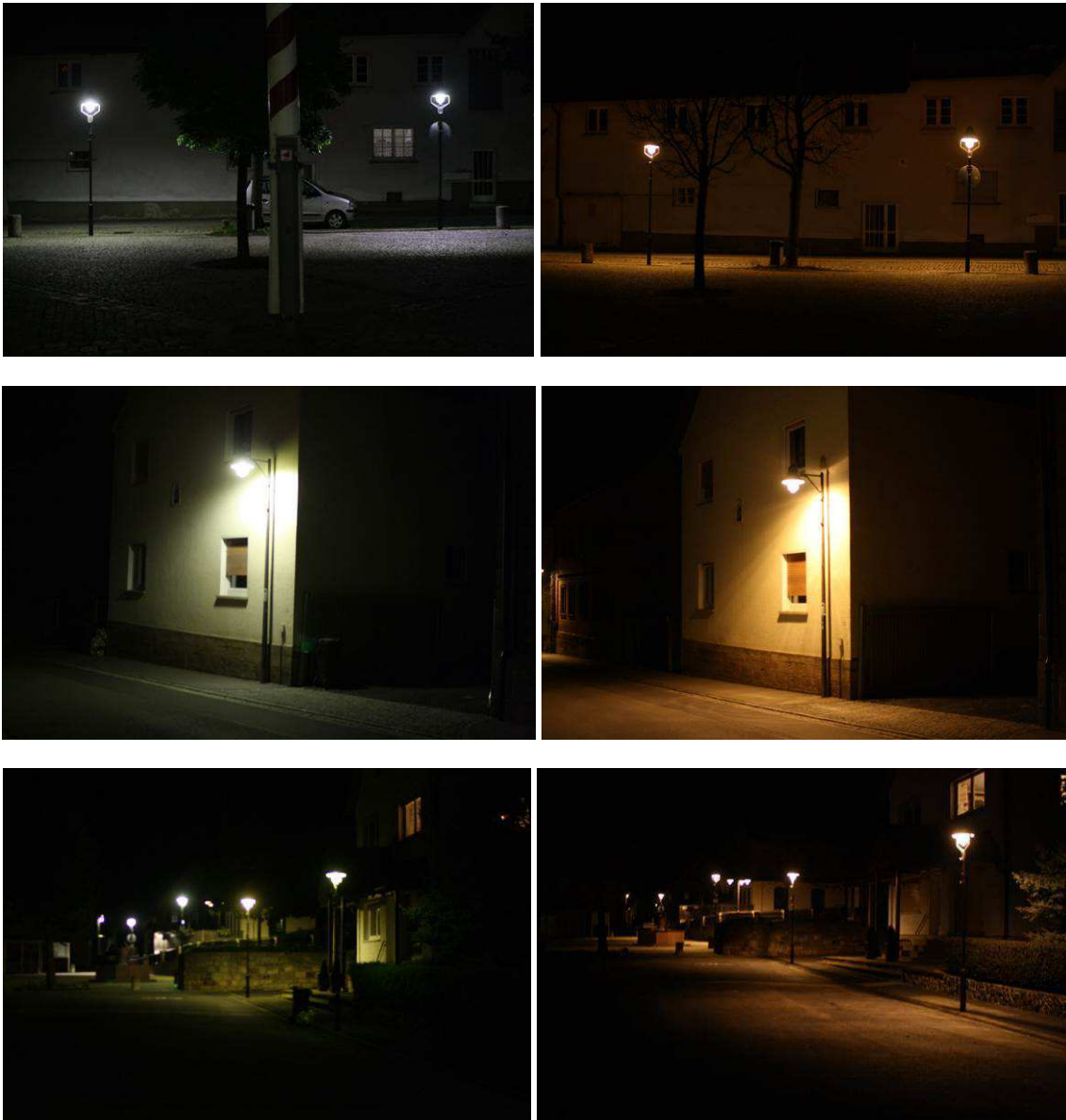
Fig. 9.7: Old HQL lighting in Oberelsbach (left side) has been replaced by 3000 K LED (right side). In the top left picture, in the right side a luminaire with a test LED kit with 4000 K was installed. The pictures on the right were taken using double exposure time (1/10 s) compared to the pictures on the left (1/20 s)
