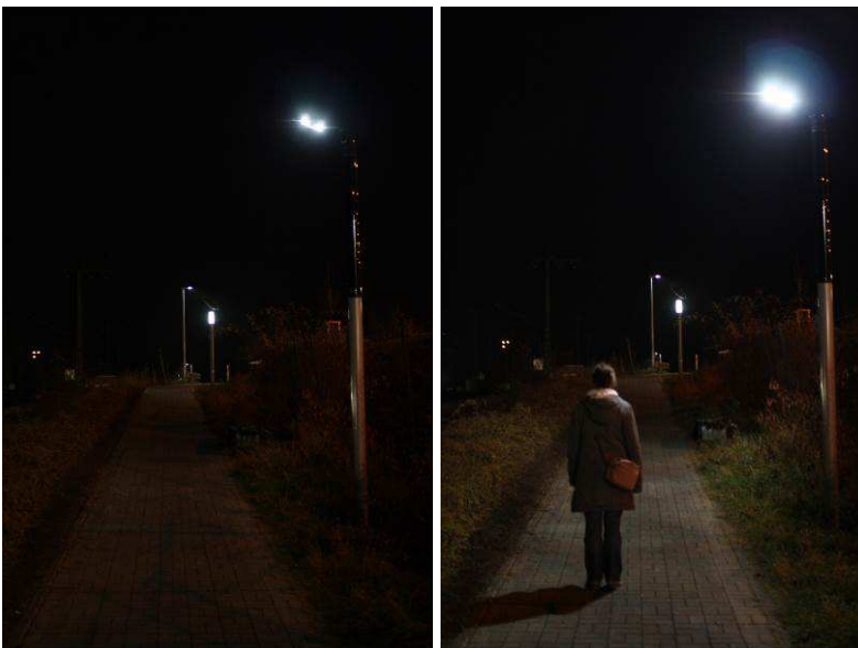
Fig. 9.20: On the left the luminaire at normal reduced light level that is turned to full intensity when a person approaches
