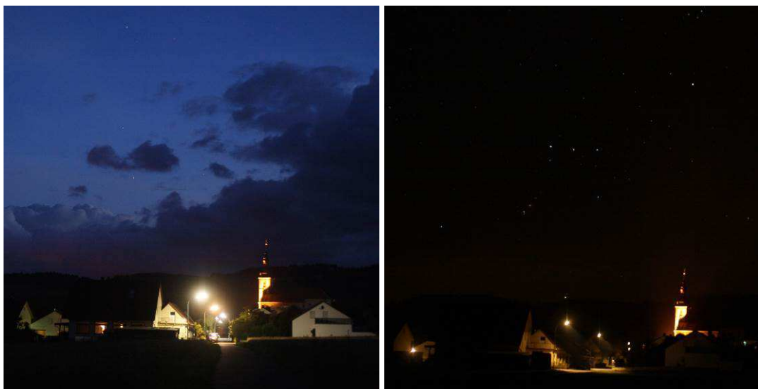
Fig. 9.8: left: Old whip luminaires with fluorescent tubes, right: new 3000 K LEDs (same exposure values!)
